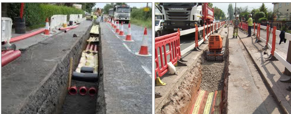
Plate 1: Typical Trenching Works set-up on the Public Road
